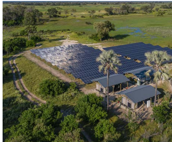
Extensive photovoltaic solar farm powered by Tesla technology ensures Xigera is entirely solar-powered
